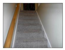
(2) Basement stairs and hand railing were in satisfactory condition. There was no railing on the open side of the stairs. For added safety, railings and or balusters could be installed.
