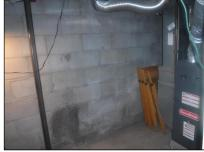
(2) White efflorescence (powder substance) on block wall indicates moisture is in contact with the masonry. This does not necessarily indicate that intrusion will occur. I recommend checking the gutters and downspout drain lines for proper drainage away from the home. Also, the grading should be pitched away from the home. Efflorescence is found on many homes without water intrusion occurring inside the home. But, it should alert you to the possibility that future steps may be needed.
