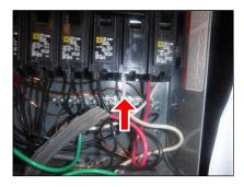
(2) One breaker was triple tapped in the electrical panel. Tandem breakers, which are rated for two wires, should be installed to accommodate multiple circuits. A licensed electrician should further evaluate and repair as needed.
