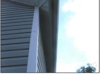
(2) There was a loose piece of soffit trim on front gable end of the house. Recommend repair as needed.
