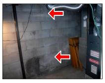
(3) The moisture meter was reading that the foundation has moisture left of the hot water heater that appears to be seeping in from the outside, possibly from the sprinkler system hitting the house. Recommend a qualified contractor further evaluate and repair.
