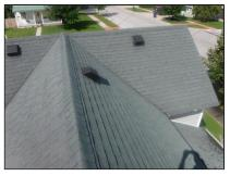
(2) Exposed nail heads and small holes on the ridge cap ends should be sealed with roof cement.
