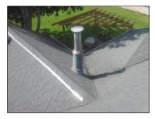
(2) The metal roof vents above roof were in satisfactory condition.
